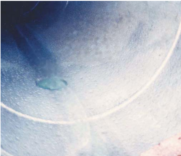
Figure 2. The pipeline once it had been cleaned.
