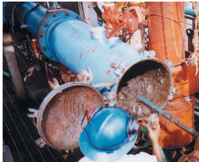
Figure 1. Removing the wax from inside the pipeline.
